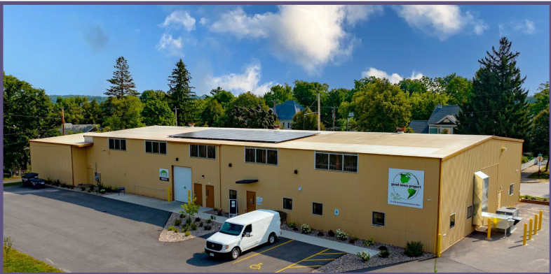
Good News Project office and warehouse get a facelift! 1106 N Fifth St. Wausau, WI
